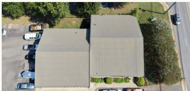
OVERHEAD — ROOF AND PARKING
